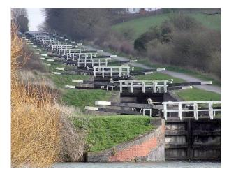
We have 1,723 km of canal, 48 canal supply reservoirs, and 97 licensable abstraction points supplying the canal network within the Water Resource West area. Typical average daily regulated abstraction is nearly 650 Ml/d (based on historical data/estimates for period 2011-17), and in addition there are considerable volumes of unregulated abstraction.
